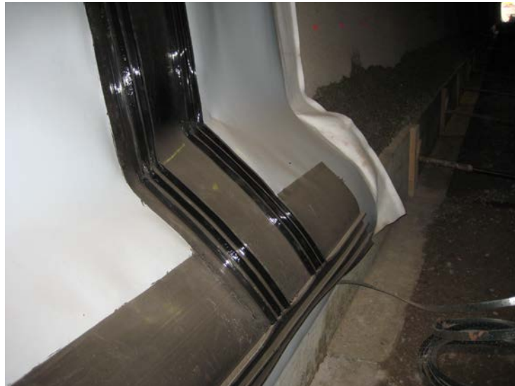
Figure: Installed water stops
