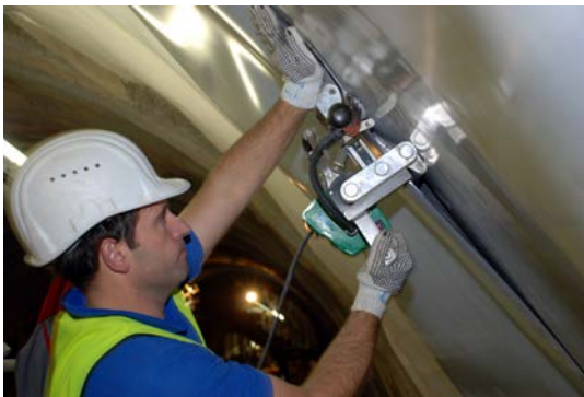
Figure: Installation of waterstops
