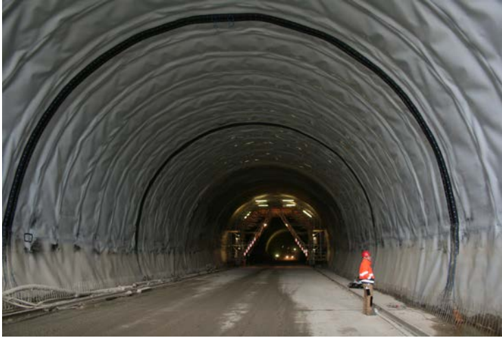
Figure: Installed waterproofing arch
